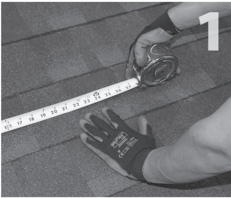
1 Choose placement of conduit mounts along path of conduit.
