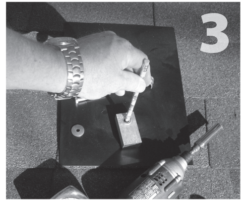
3 Slide conduit mount into desired position. Remove any nails that conflict with getting the mount flush with front edge of shingle course. Mark center for drilling.
