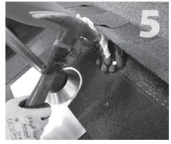
Under the 3rd course and through the 2nd course, secure flashing with 2 roofing nails at the top corners of the flashing at the nail line. Apply sealant over nail heads.
