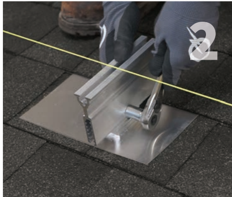
2 The string acts as a guide for aligning the top slider positions of all the mounts in the row. To adjust top slider height, remove machine bolt, separate top slider from QBlock slider and reinsert at proper location.
