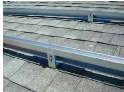
Fig 9.1 - Standard rail mounting
