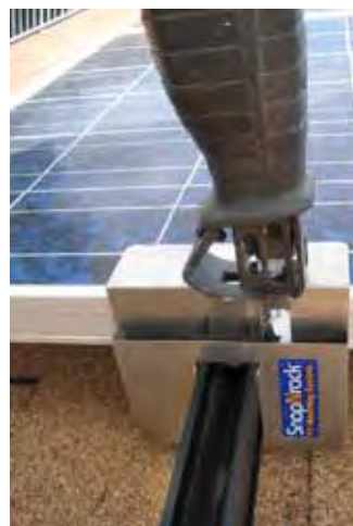
Figure 2.3 UEC Rail Cutting Guide
