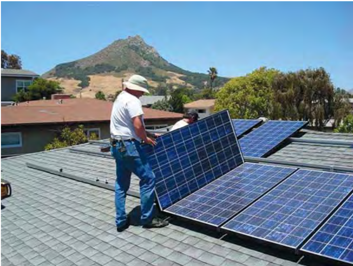
Figure 1.0 - Placing modules on S100 standard rails installed on L-Feet
