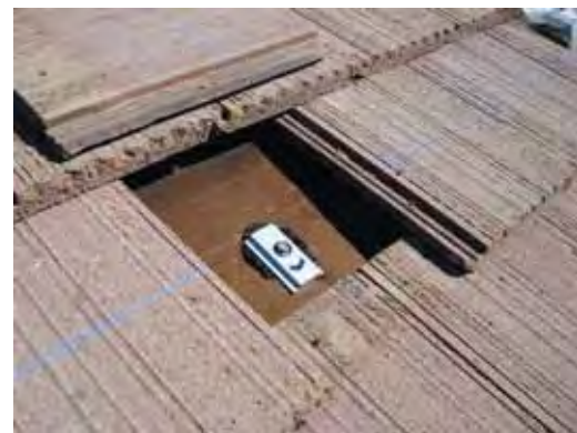
Typical standoff base installation
