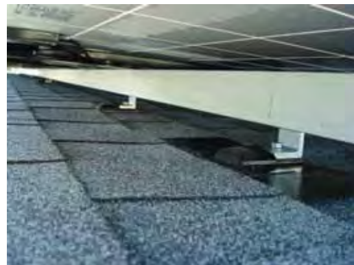
Check under the array for dangling wires
