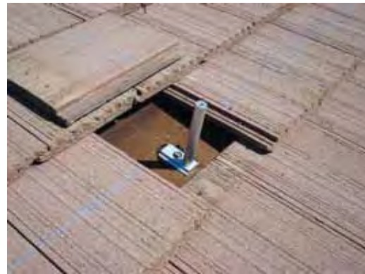
Screw standoff onto base
