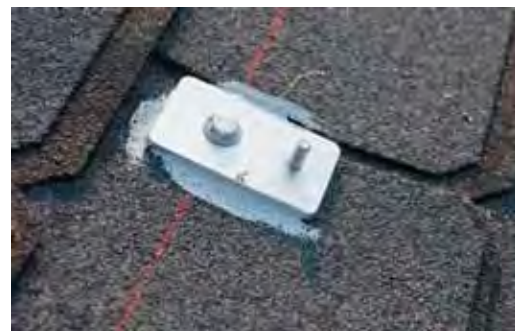
Secure base to rafter
