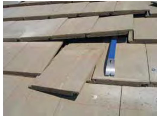
Remove roofing material to expose roof underlayment
