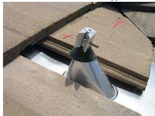
Slide standoff clamp and hardware
