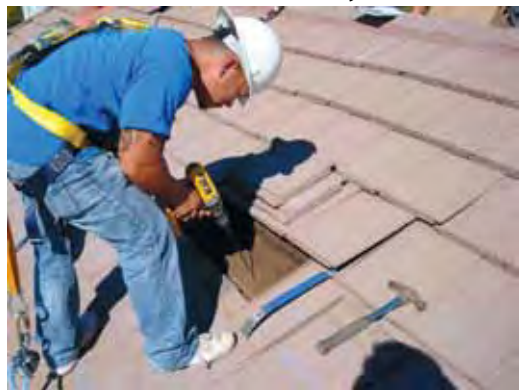
Drill pilot holes
