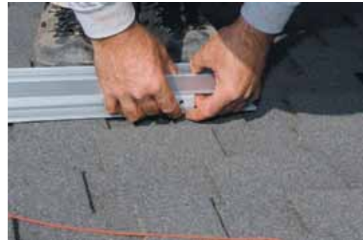
Fig 9.0 - Snap in channel nuts
