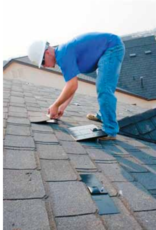
Install Flashing
