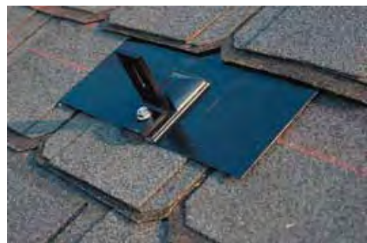
Completed Flashed L-Foot
