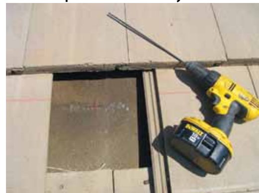
Transcribe layout lines from roofing material to underlayment
