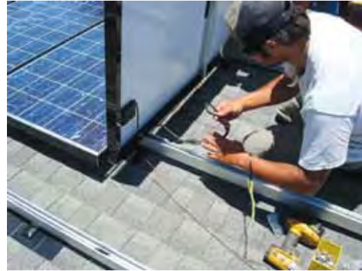
Connect wiring
