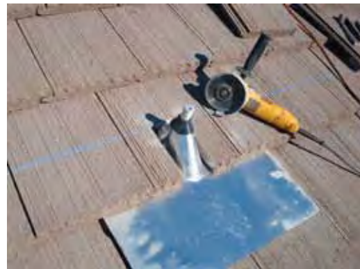
Install flashing using appropriate methods for roof type.
