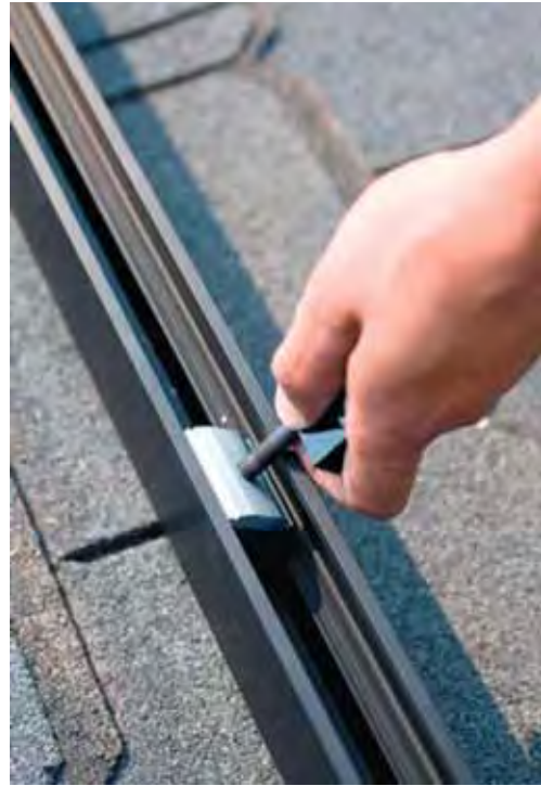
Fig 10.4 - Snap Mid Clamp Assembly into Rail
