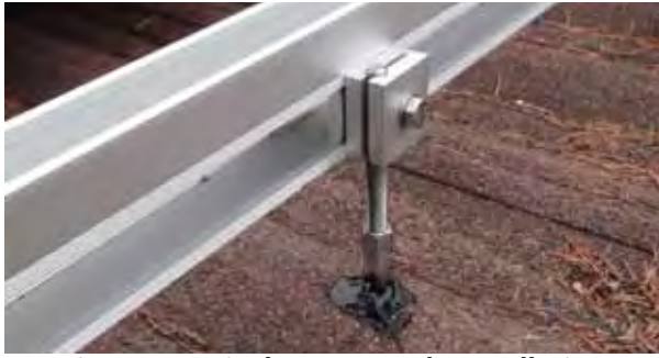
Fig 5.0 - Typical Hanger Bolt Installation
