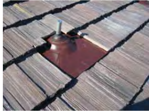
Fig 4.2 - Standoff installation using Oatey flashing
