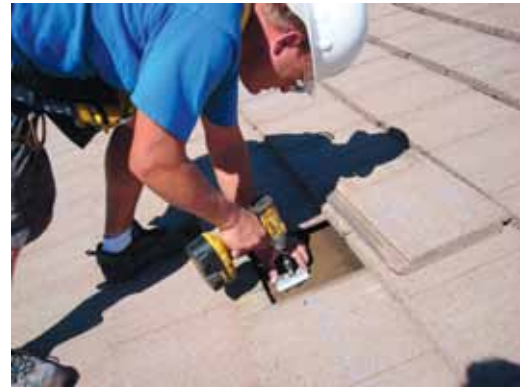
Secure standoff base to rafter
