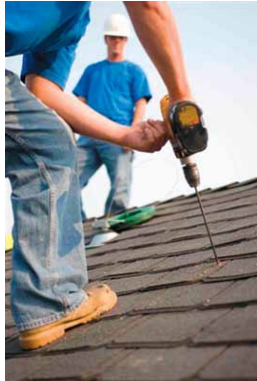
Fig 3.2 - Drill pilot holes
