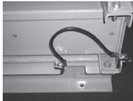
Figure 3: Cable Assembly Installation
