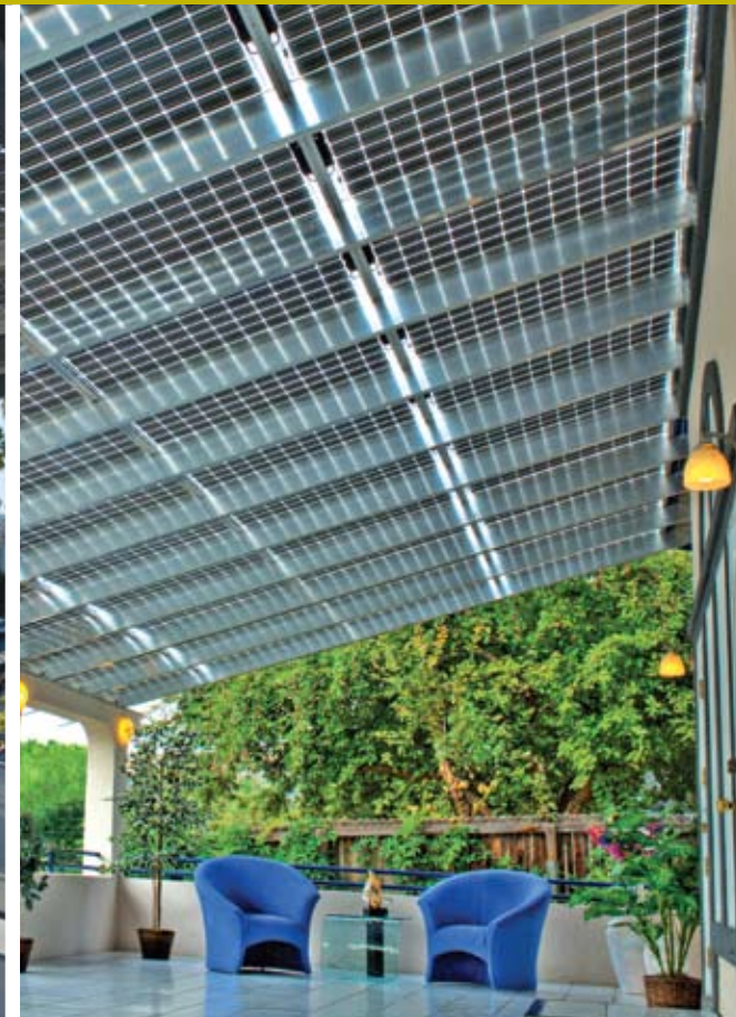
Patio Awning: 11.4kW Solar Living Design Lakewood, CO
