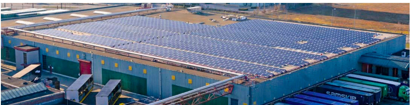
Heineken Wierckse Brewery - 921kW - 855,000kWh/year - 3,683 REC Solar Panels - Den Bosch, Netherlands
